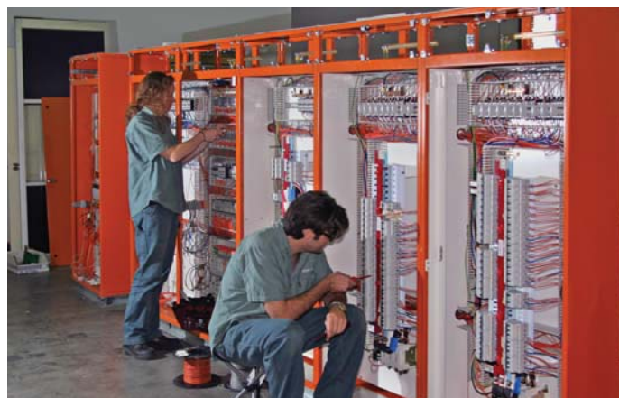
Cross-Tunnel Panels being assembled for the Clem Jones Tunnel
