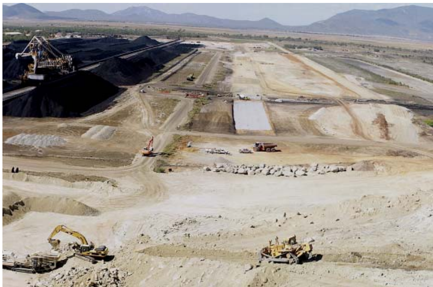
The site for the Abbot Point X50 Expansion facilities
